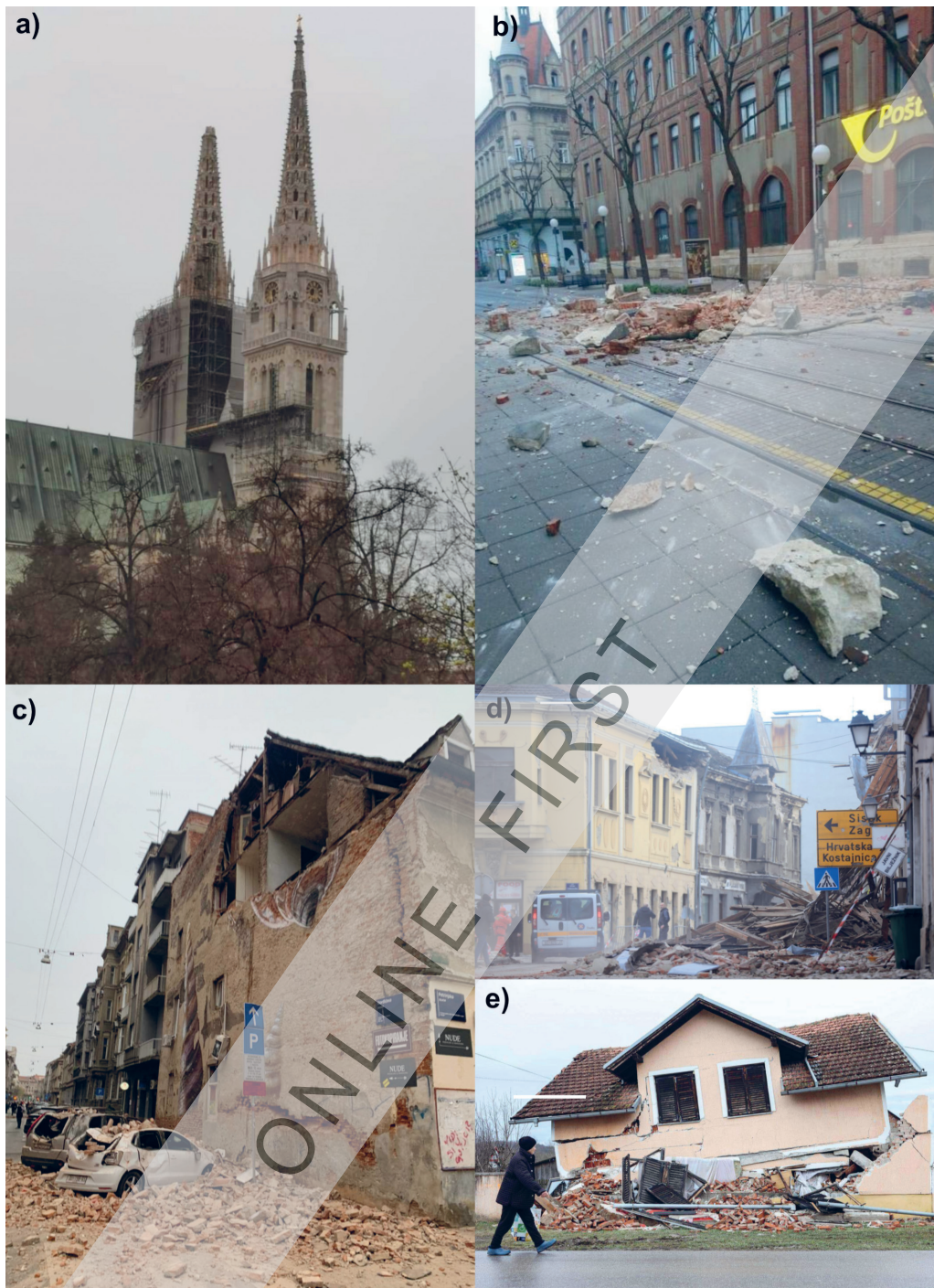
Figure 2. Some examples of earthquake damage from 2020 (Croatia): a Zagreb cathedral – broken tower top; b Zagreb main post office; c Zagreb old town; d Petrinja city – main street area; e Petrinja city wider area – collapsed family house.
